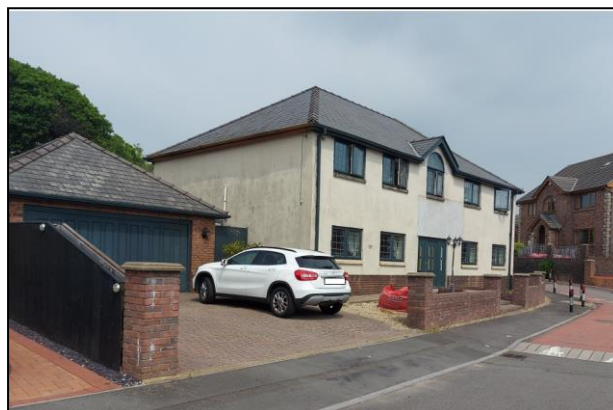
Figure 2 Photograph of existing front elevation
